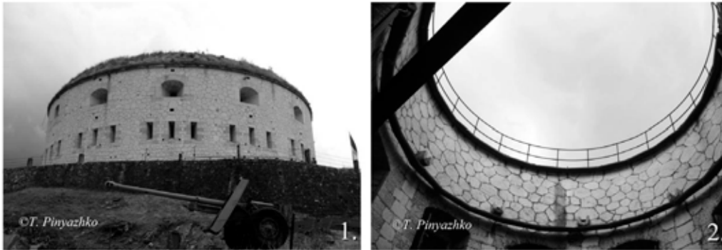
Fig. 8. Rivoli: 1. – fort Wolgemuth and the tower; 2. – internal view of the towers courtyard. Photo's 2011.
