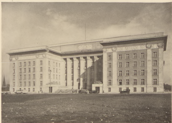
V.—KATOWICE: OFFICES OF THE SILESIAN COUNTY COUNCIL
