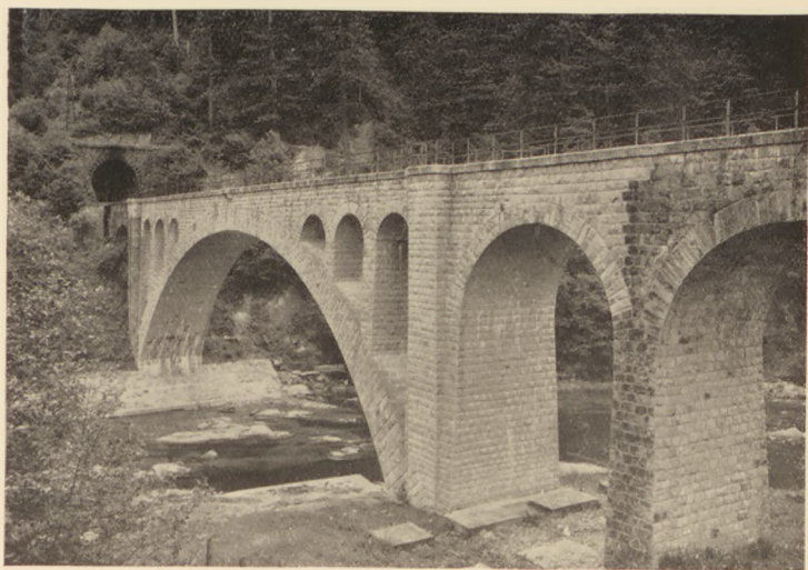
X.—RAILWAY BRIDGE AT JAMNA
