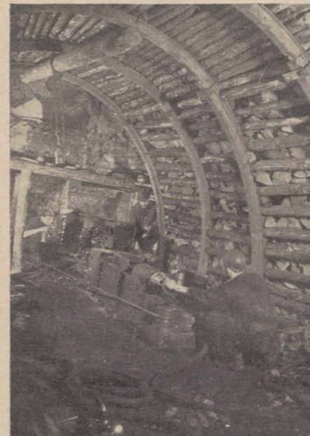
Lining up a coal cutter
