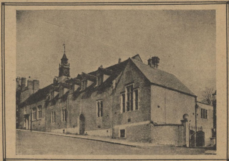
NEW SECONDARY SCHOOL, MARKET HARBOROUGH
