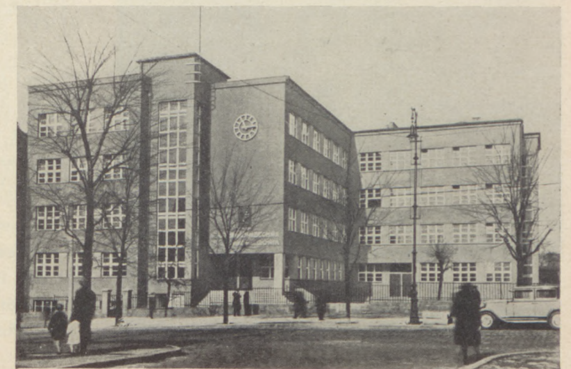
A TYPICAL MODERN HIGH SCHOOL IN POZNAN
