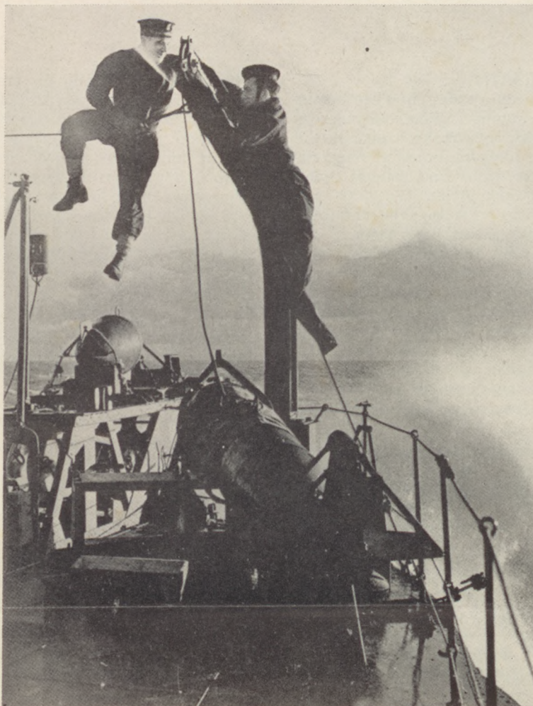
REPAIRS AT SEA
