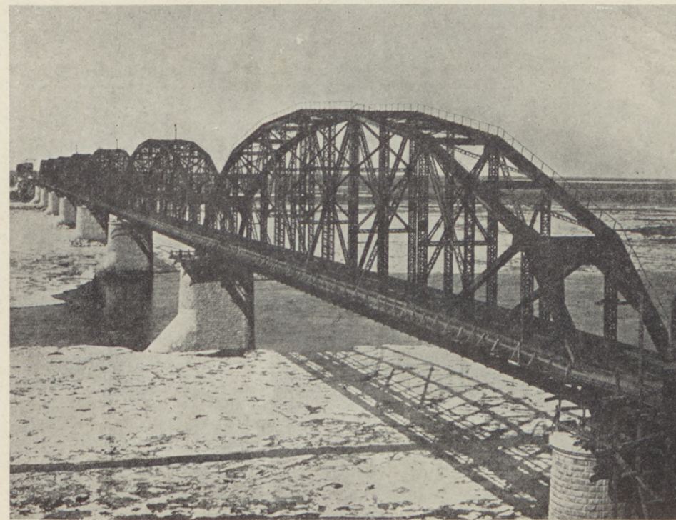
The longest bridge in the Old World, crossing the River Amur near Chabarowsk (Siberia) constructed by Messrs. "K. Rudzki and Co.", Warsaw, in 1904-1905.
