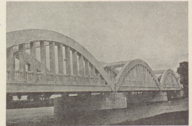
THE FIRST WELDED-STEEL BRIDGE IN THE WORLD The Bzura River bridge in Poland constructed entirely without rivets and with all parts welded.
