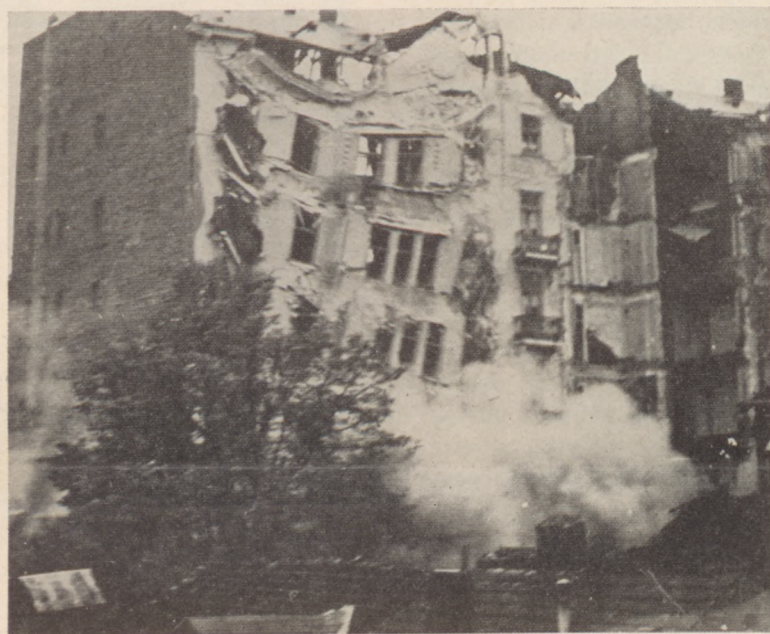
... HOUSES FELL, BURYING PEOPLE IN CELLARS AND SHELTERS ...
