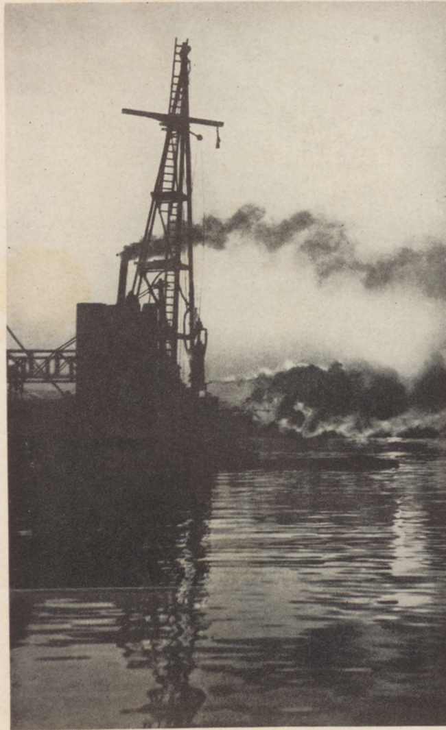
DRIVING PIER PILES
