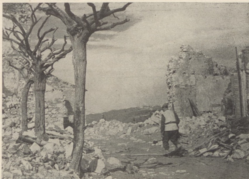
During winter weather Polish sappers helped to clear roads of the deep snow to enable troops and transports to go forward. Here is part of a village which the Germans demolished before retreating.
