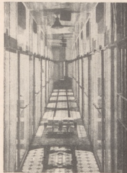
Vault of Bank Polski, Warsaw.
