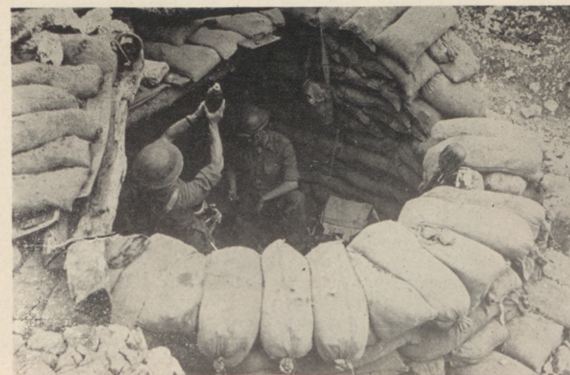
Polish mortar gun site. Polish Second Corps in Italy.
