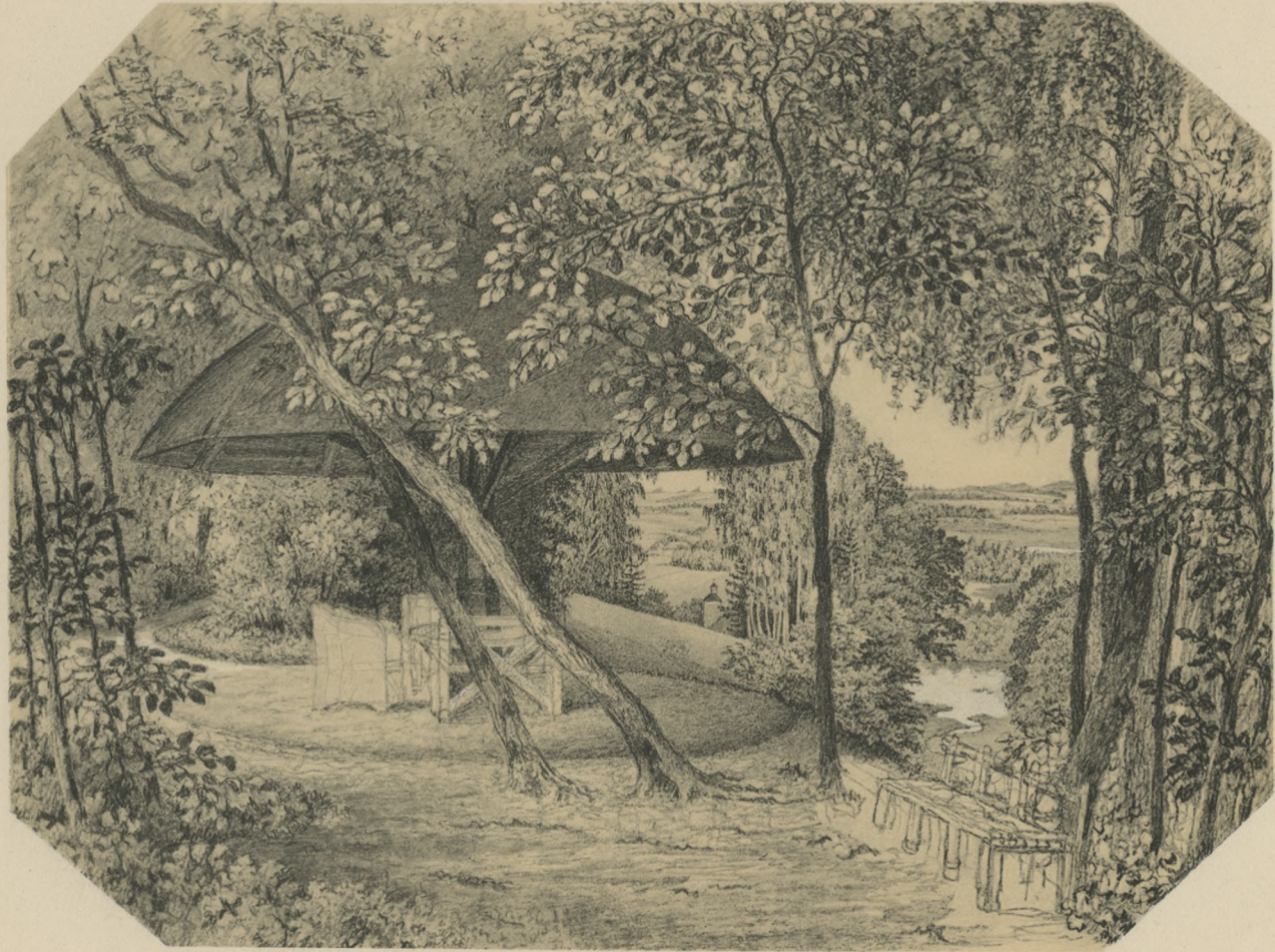
W. S. Stavenhagen Heimthal in Livland September 1857
