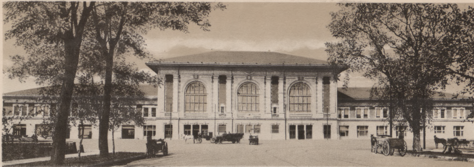
DENVER, RIO GRANDE AND WESTERN PACIFIC UNION DEPOT.
