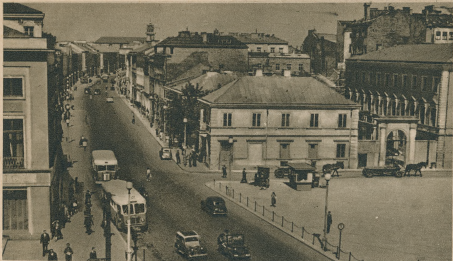
The complete reconstruction of Nowy Swiat has restored the historical architecture of the damaged buildings.
