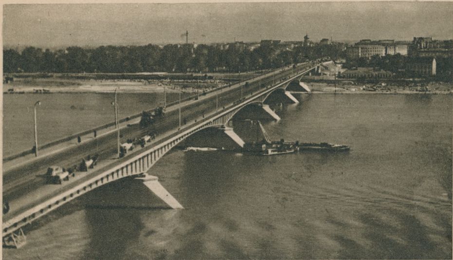
The newly constructed Śląsko-Dąbrowski bridge, a part of the modern East-West Highway. 1950
