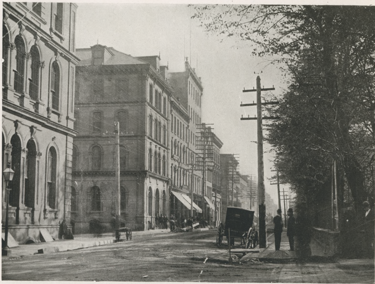
HOLLIS STREET, LOOKING SOUTH FROM THE POST OFFICE
