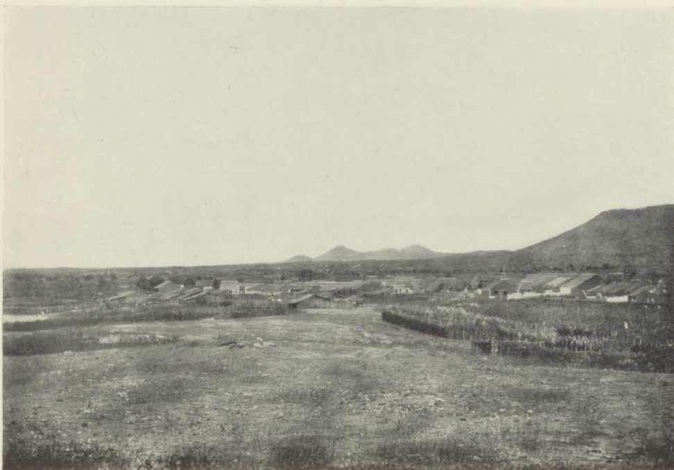
Phot. Inspect. de Obras contra as seccas.
