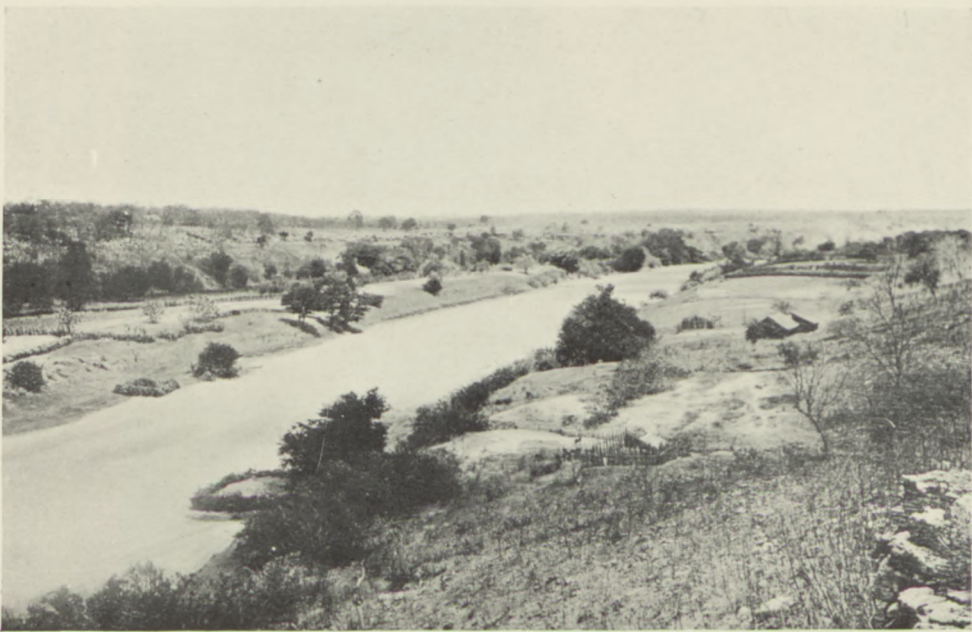
Phot. Inspect. de Obras contra as seccas.
