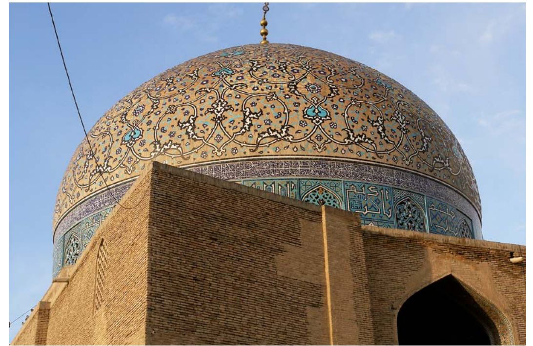
III. 1. Masjid-i Sheikh Lutfallah. The Dome outside ceramic decoration. Kashi-ye mo'arra (cut-tile mosaic or inlaid tiles); phot. Vadim Pappe
